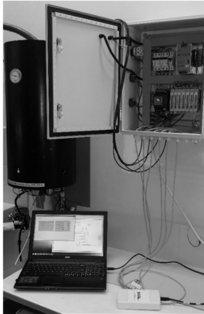
Fig. 1. Experimental set-up to research inductive heating of domestic hot water
