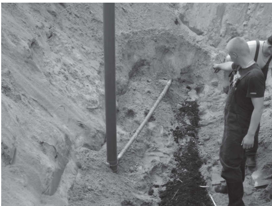
Rys. 10. Piezometr wraz z fragmentem bariery Fig. 10. Piezometer with drainage and part of compost barrier
