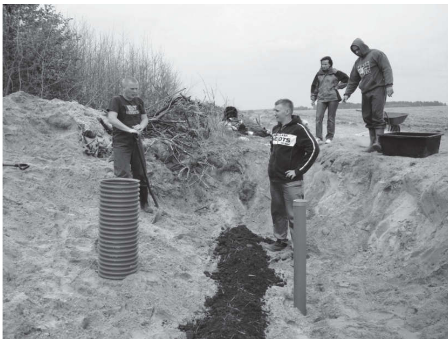
Rys. 11. Widok na fragment bariery Fig. 11. View of a barrier
