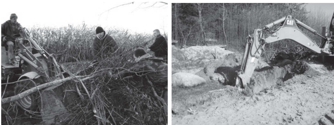
Rys. 7. Oczyszczanie terenu mogilnika. Praca koparki na terenie mogilnika Fig. 7. Refining of graveyard area. Excavator near graveyard
