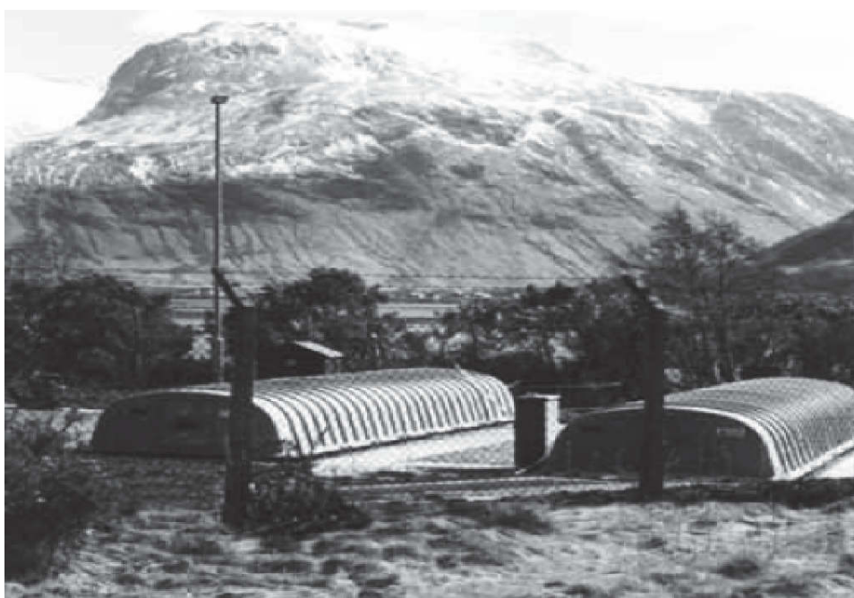
Rys. 5. Oczyszczalnia z TZB – Corpach, Anglia Fig. 5. The wastewater treatment plant RBC – Corpach, United Kingdom
