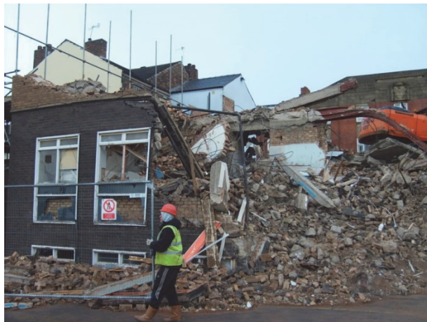
Fig. 1.1. Exemplary European demolition site (photo by J. Katzer)
