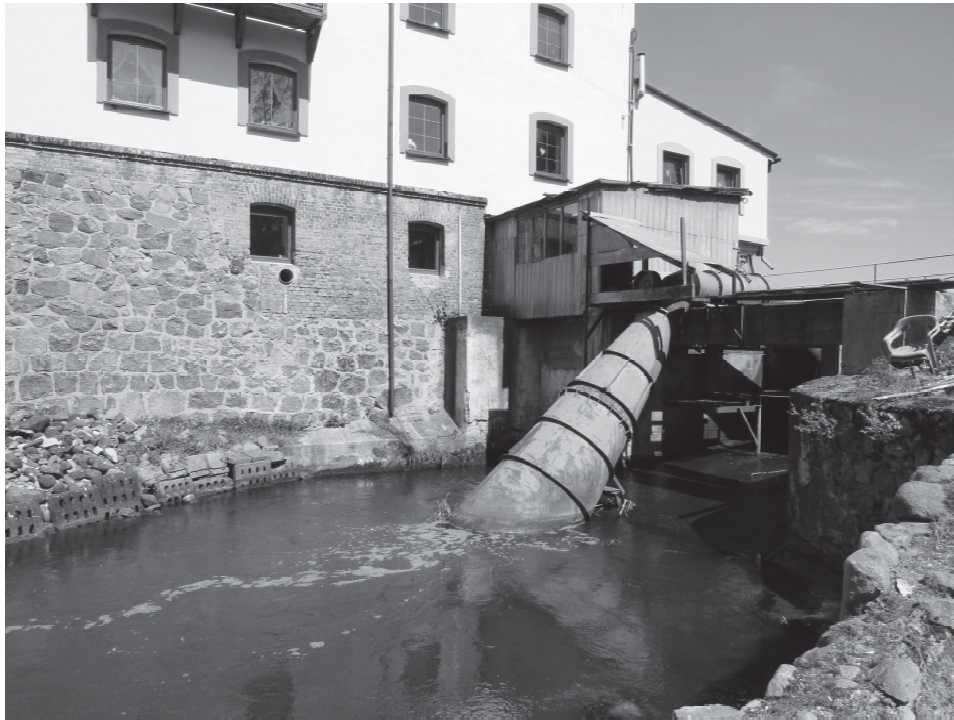
Fig. 4. Downstream view of SHPP at the Dobrzyca barrage on the Głomia river
