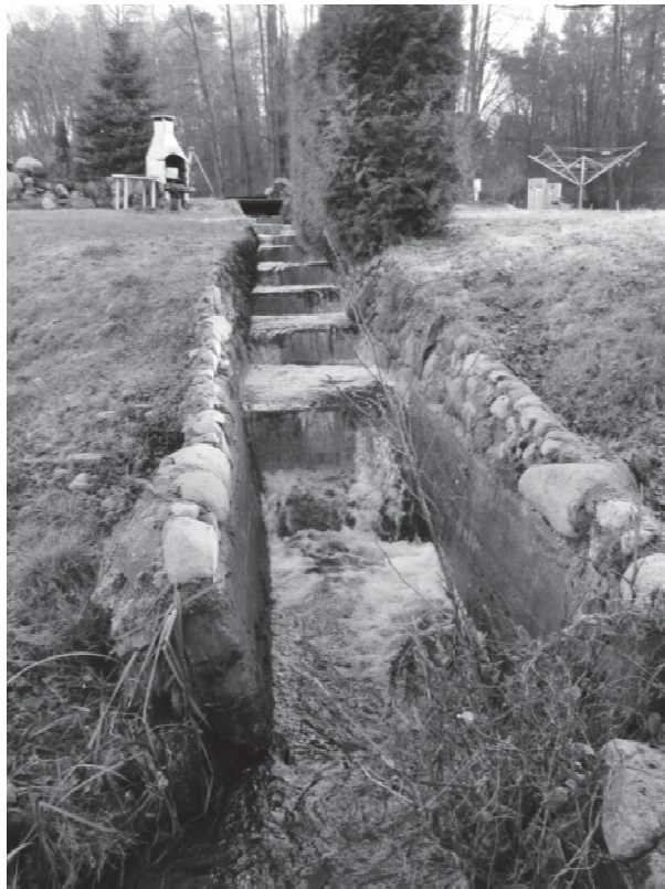
Fig. 5. Pool fish pass by Dobrzyca barrage on the Głomia river
