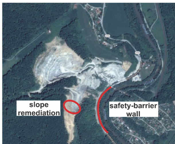
Fig. 2. Schematic representation of the slope remediation and safety-barrier wall (EU-ROVIA – Kameňolomy, s.r.o. Košice 2017)
