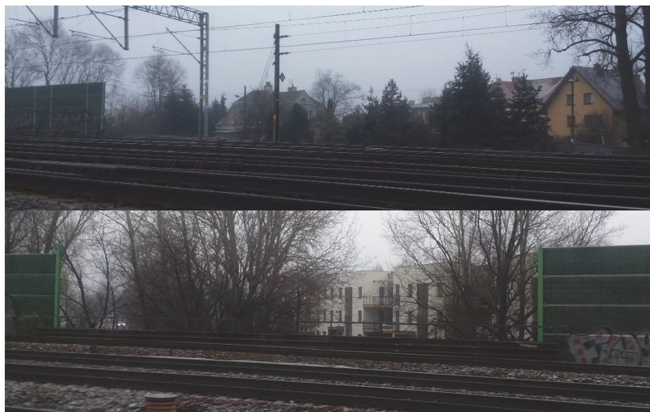
Fig. 5. The discontinuity of acoustic barriers [autor's photo]
