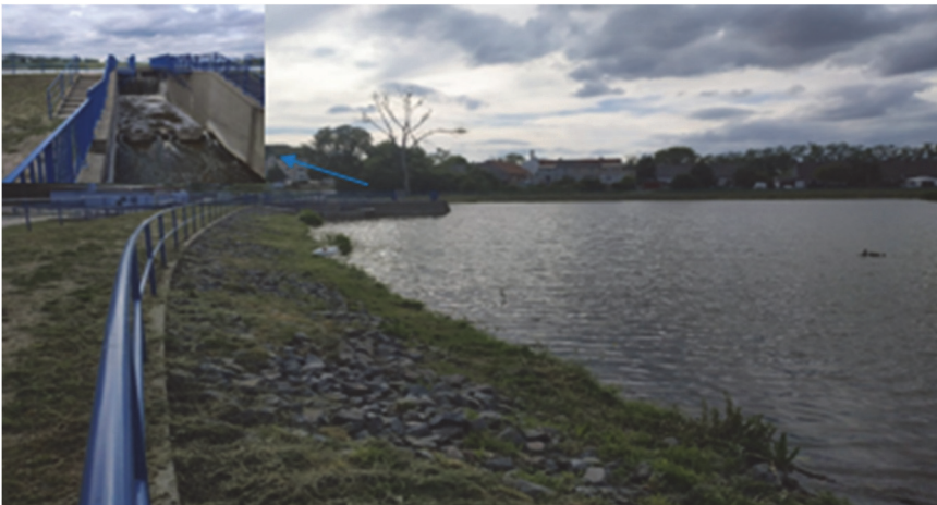
Fig. 2. The embankment dam with the spillway-overflow structure (steady level damming) in the Przebédowo reservoir
