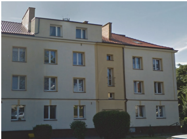
Fig. 1. Multifamily building with analysed apartments
