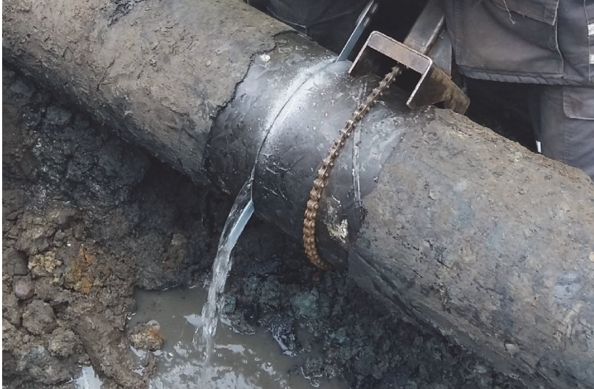
Fig. 1. Cutting of the DN300 gas pipeline at Myśliwska in Kołobrzeg
