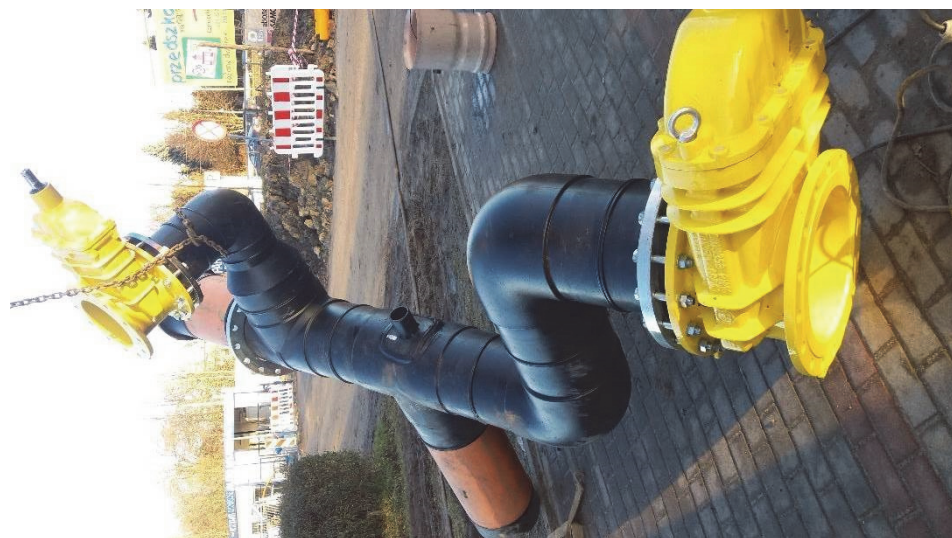
Fig. 3. Polyethylene dehydrator with diameter DN 355 (without inspection pipe)
