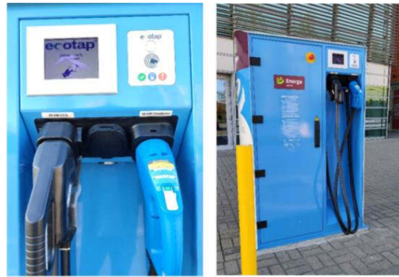
Fig. 9. 50 kW charger at the EMKA gallery in Koszalin
