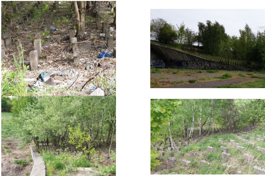
Fig. 2. Current stadium status
