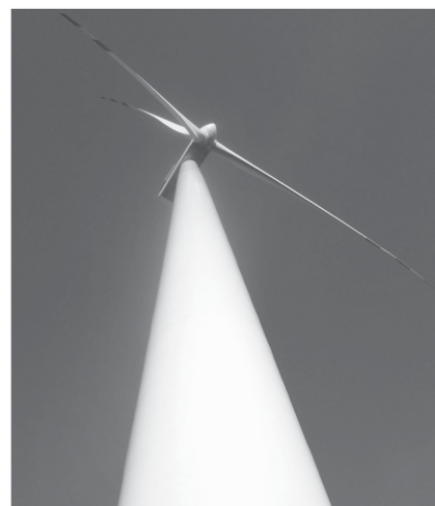
Fig. 2. Analyzed turbine with a tubular tower.
