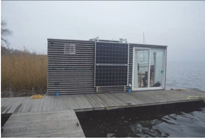
Fig. 1. Example overview of water house (WH) moored to the bridge at the lake quay – view from the entrance to the building (own materials)
