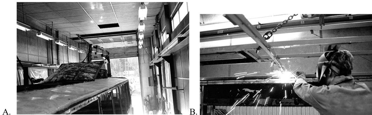
**Fig. 9.** A – Removal of the roof using a crane or overhead crane; B – Removal of bumpers, all flaps and roof framing
